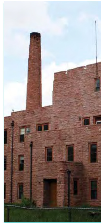
Original Ft. Defiance Indian Hospital
